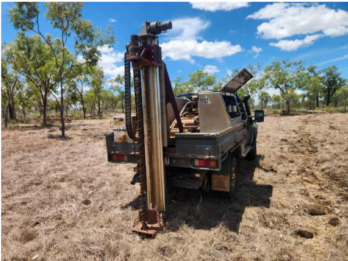
Site testing at 50186 Gregory Development Road, Greenvale.
