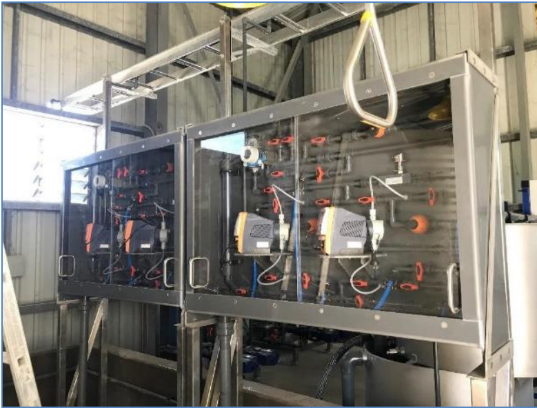
Figure 3-7: PolyDADMAC Dosing Panels
