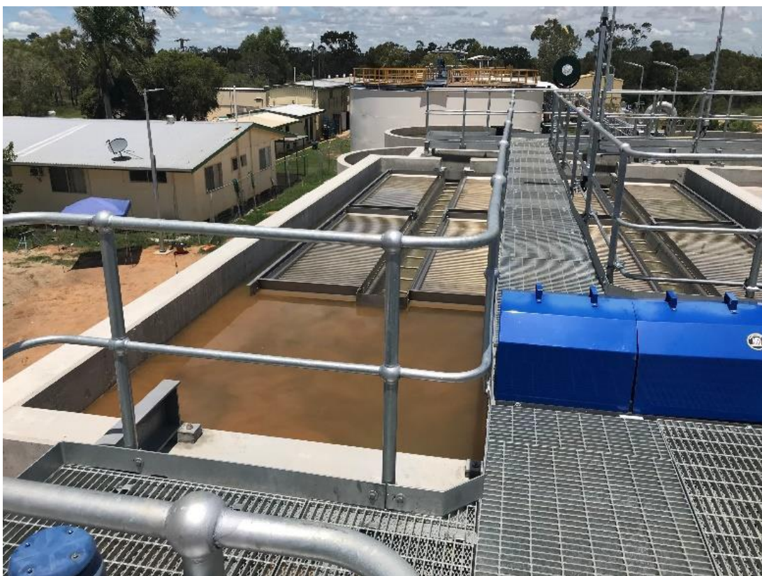
Figure 3-5: Clarifiers and Lamella Plates
