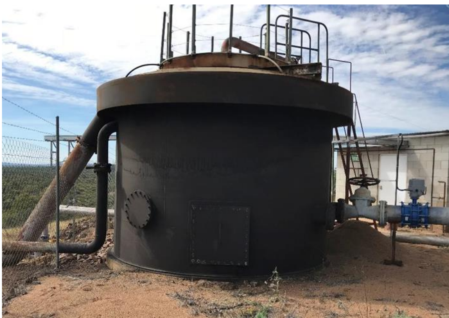
Figure 3-13: Greenvale contact tank
