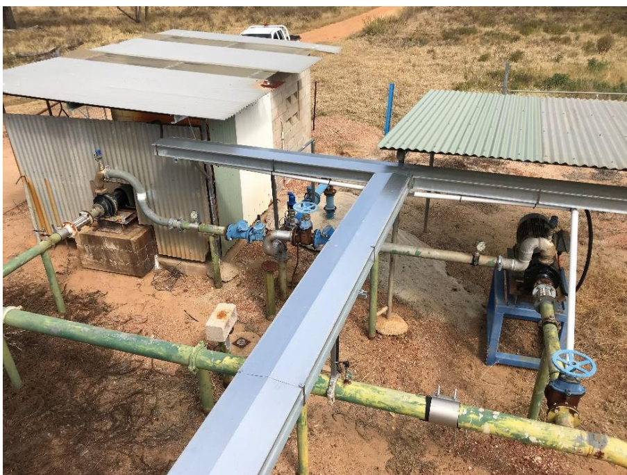
Figure 3-12: Greenvale bores lift pump station
