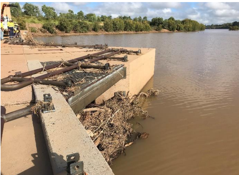
Figure 3-3: Trash Accumulation at Weir Intake after Flood Event
