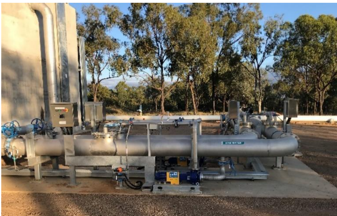
Figure 3-4: Plant inlet and dosing
