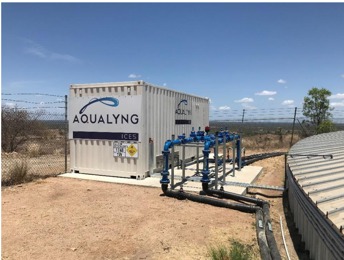
Figure 3-10: Re-chlorination system at Towers Hill Reservoirs
