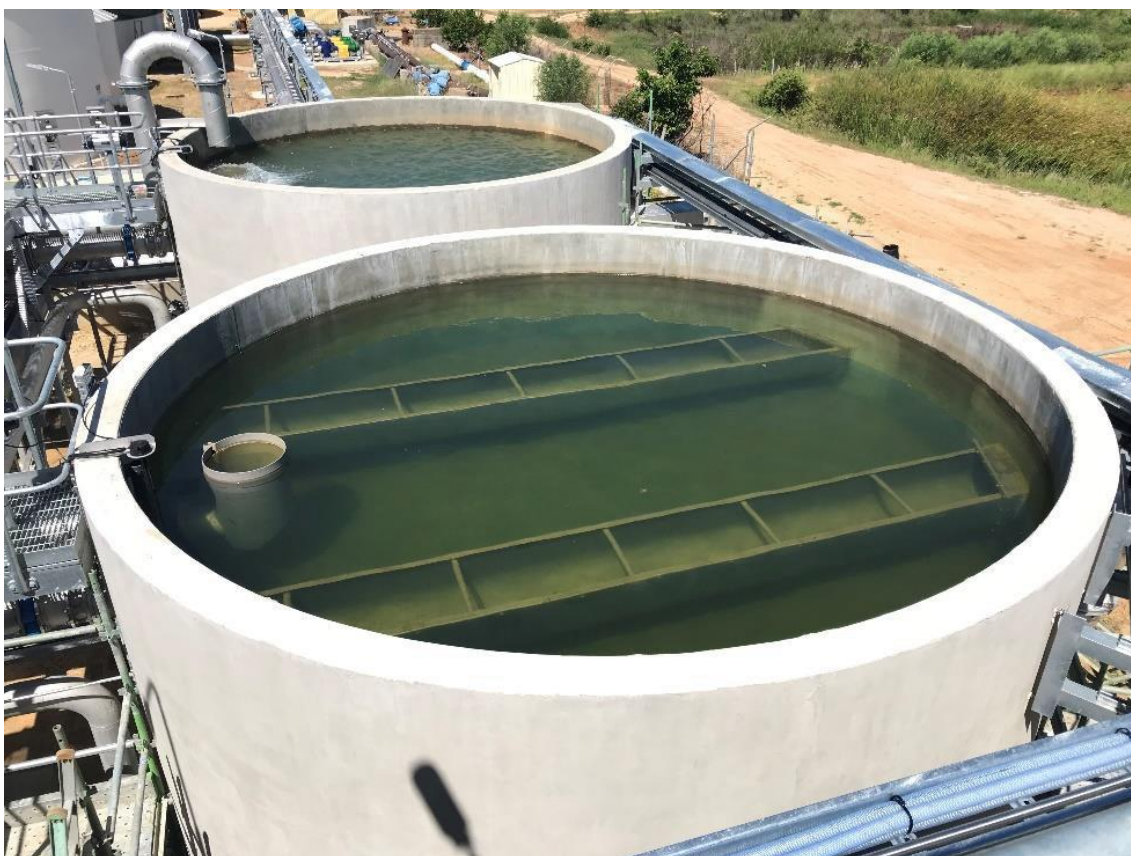
Figure 3-6: WTP Gravity Filters
