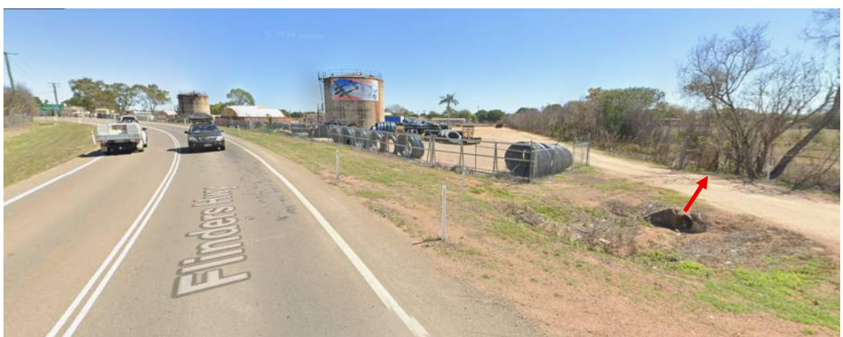
Figure 4.2 - Site Exit - Culvert Under the Driveway and Discharging Into the Adjacent Lot (Google Maps)
