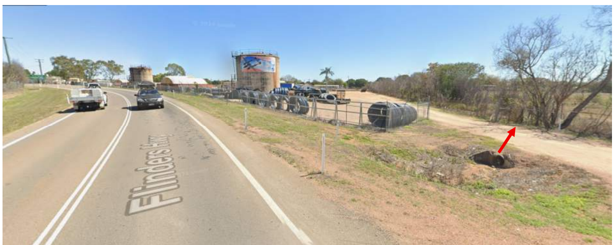
Figure 4.2 - Site Exit - Culvert Under the Driveway and Discharging Into the Adjacent Lot (Google Maps)
