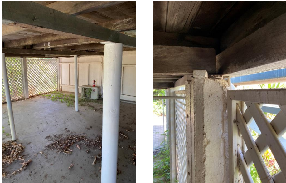
Figure 5: Concrete Post with No Identifiable Fixing
