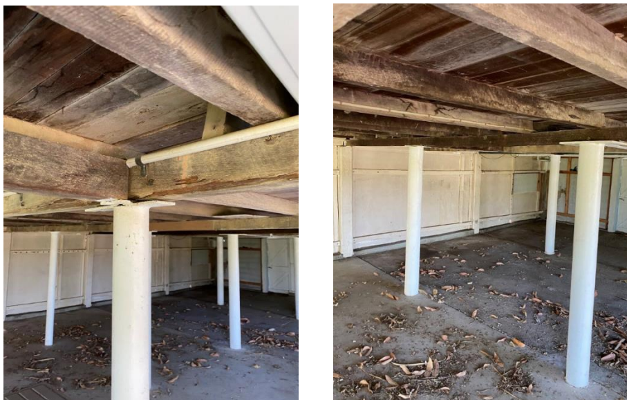
Figure 3: Timber Floor Framing
