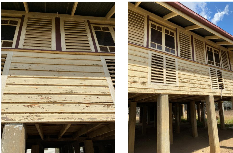
Figure 4: Deteriorated Cladding
