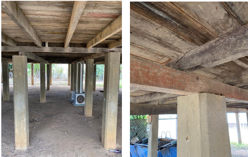
Figure 3: Timber Floor Framing
