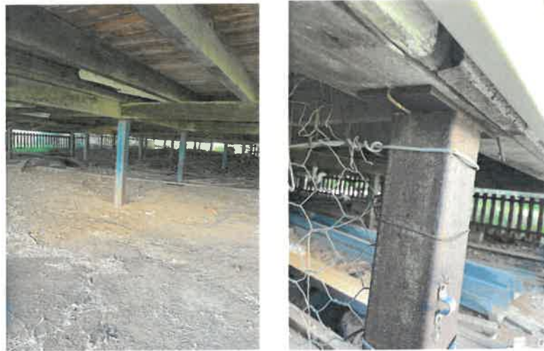
Figure 4: Timber Floor Framing
