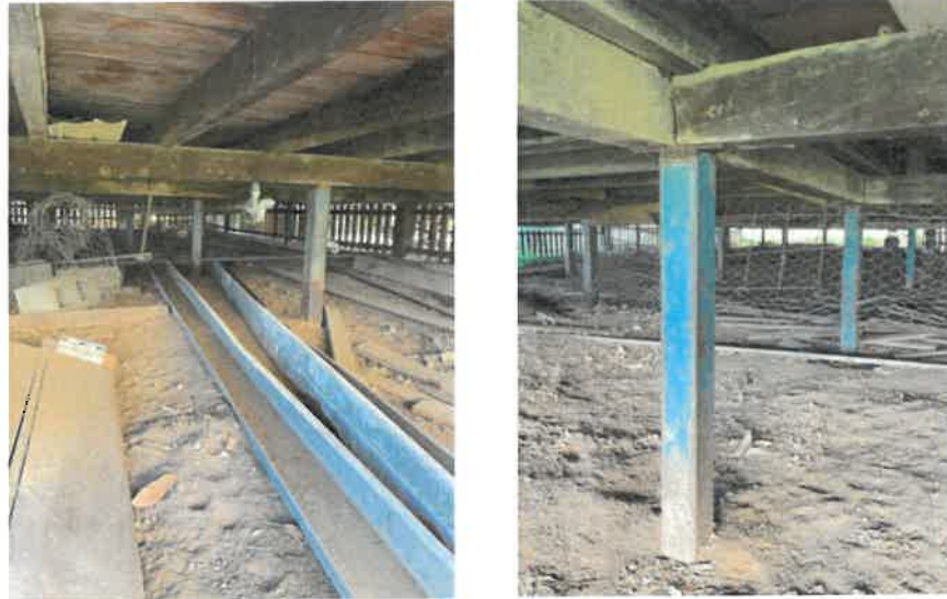
Figure 3: Posts supporting timber floor framing.
