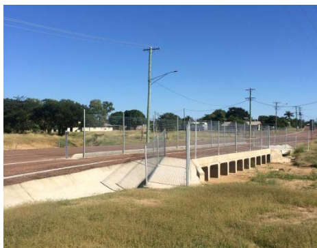
Culvert installation - Buchanan Creek at Brisk Street
