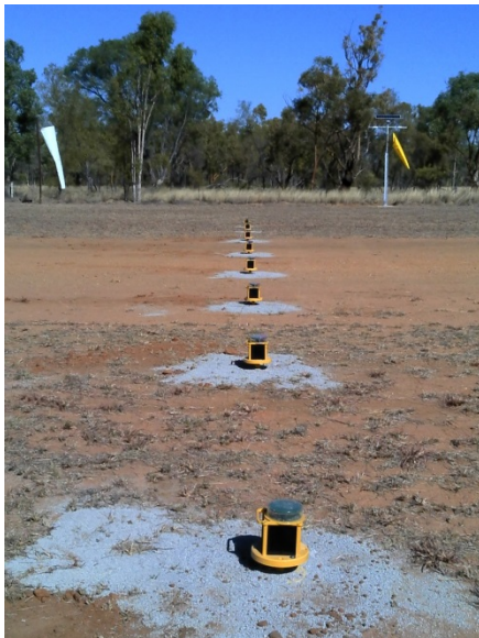
Solar lighting at Pentland Airstrip
